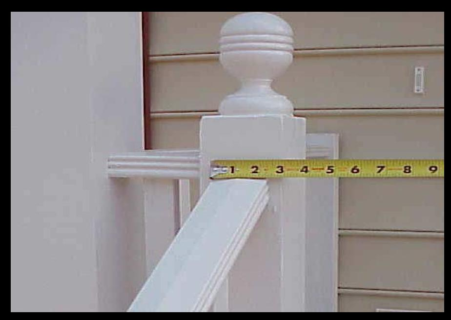
THIS HANDRAIL PROVIDES EQUIVALENT GRIPPING AREA
