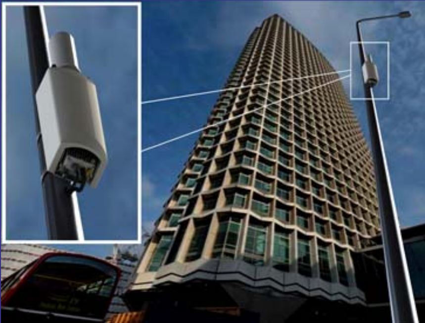
Small Cell Facilities – 6 SF or less
